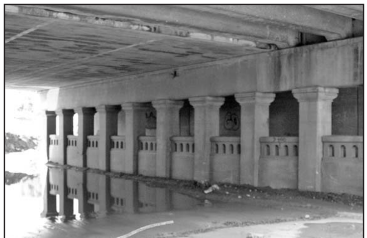
August 26, 2010 one last photo of the Robinson Avenue bridge. About 2/3's of the bridge has been removed
